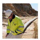
Washed gold bearing slurry from old re-worked slimes dams was needed to be piped 52 km to processing plants. The piping system included 2 pump stations with 10 pumps in series.
