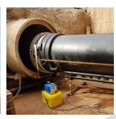
Mocke Pipelines installed 1200 mm diameter HDPE pipes, SDR 21 with a wall thickness of 57.2mm at Medupi Power Station.
